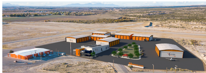
Tech1 Campus-Alpha Site Fabens, Tx
